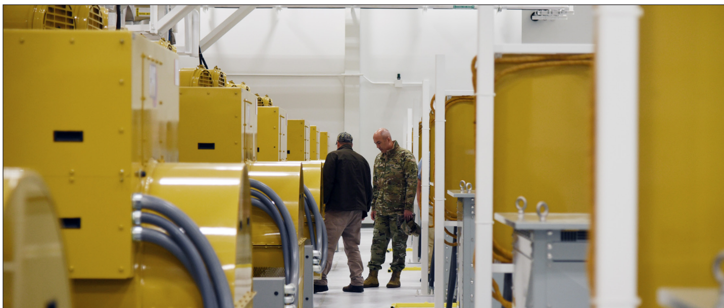
Mike Doty, Alaska District electrical engineer, takes Col. Sebastien Joly, Huntsville Center commander, on a tour of the generator room in the Long Range Discrimination Radar power plant at Clear Space Force Station, Alaska. The power plant houses generators as a back up energy source to keep the radar active in case of power failure.
